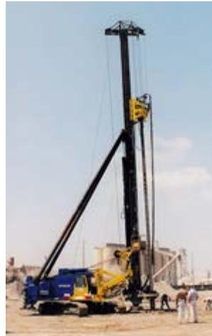
The construction of seven new GE combustion turbines and heat recovery steam generators at the existing Tampa Electric Company (TECO) Bayside Plant in Tampa, Florida required foundations to meet extremely tight total and differential settlement criteria. The subsurface geology comprised a variable sequence of very soft silty and clayey soils overlying a pinnacled weathered limestone.
