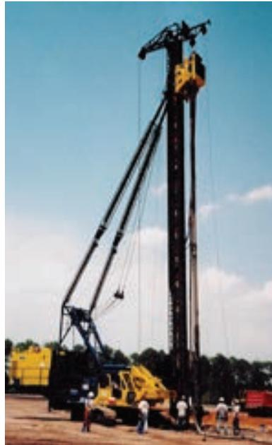
The construction of the new Oleander Power Facility in Cocoa Beach, Florida required a deep foundation system. Four turbines, stacks, pipe racks and support structures were to be constructed over very soft silts and clays extending to depths of up to 45 feet below grade. Preliminary recommendations included precast piles or augercast piles. The project base bid foundation ultimately comprised 18-inch augercast piles 75 feet in length, with design loads of 40 tons.
