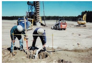
The 405 16" diameter CFA piles used in the moderately loaded structure areas, were installed by a similar Hitachi base machine with a high torque hydraulic turntable.
