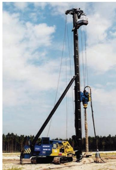
In areas of deep overburden, where high loads were present, cased ahead drilled shafts were used. This system uses a sectional casing to stabilize the bore as the soil and rock is drilled out and stockpiled. Upon reaching the required depth, the reinforcing cage is installed prior to concrete being placed via a tremie.
