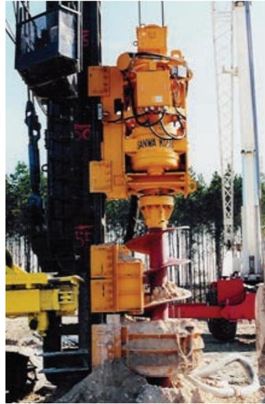
crane fitted with a high torque mast and electrical turntable. With this system, a 1-meter diameter hollow stem auger is advanced to the required depth, prior to grout or concrete being pumped under pressure as the auger is withdrawn without rotation using 120-tons of line pull. The grout forms a monolithic column into which a reinforcement cage is inserted.
