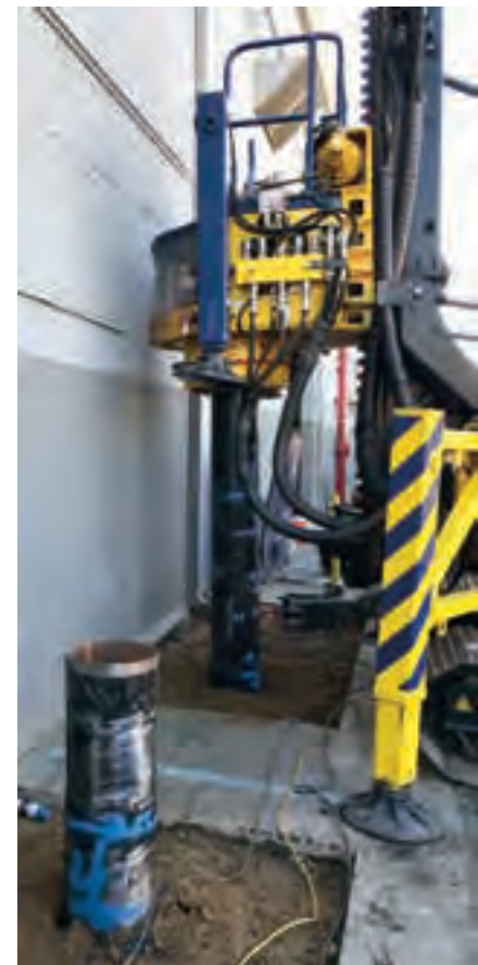
Installing PC-CIDH pile in tight space near exterior wall
