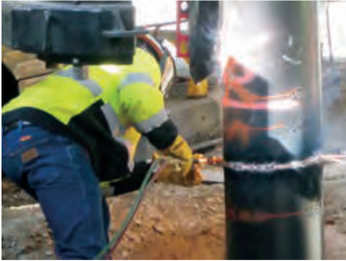
Welding additional casing length on PC-CIDH pile
