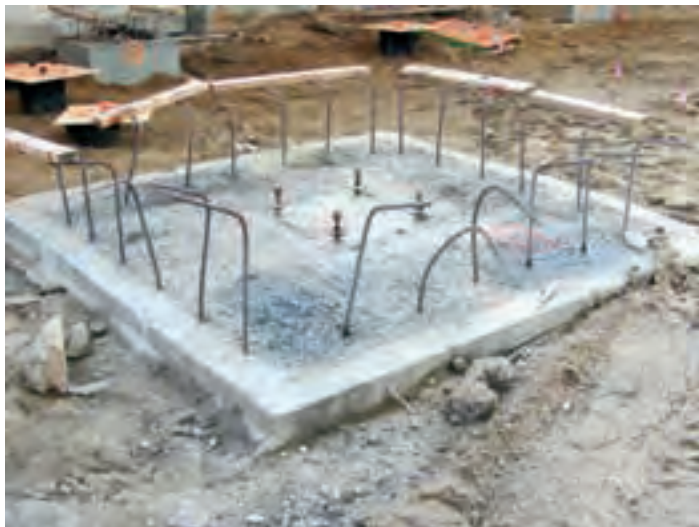
Constructed pile cap atop PC-CIDH piles
