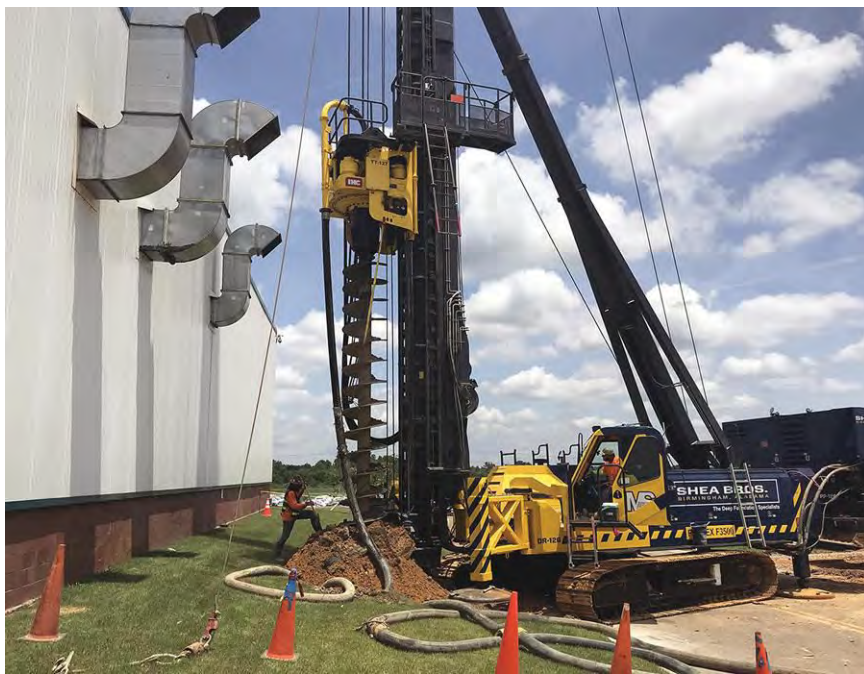
1-m-dia CFA piles are installed on a project in Montgomery, Ala.
